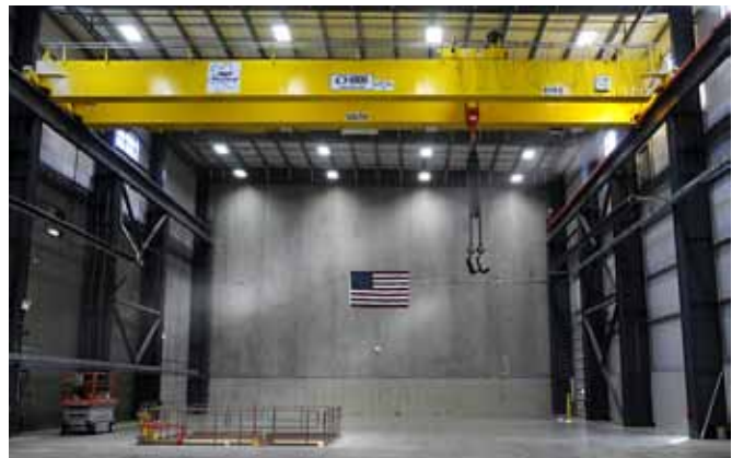
This 100-ton crane provides unique fabrication capabilities at AT&F's nuclear facility.
